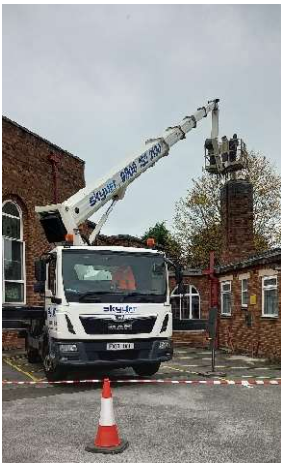
The new flue being installed
